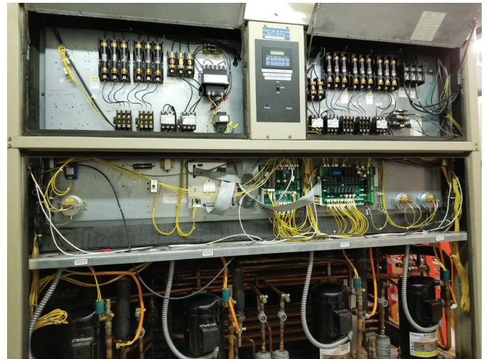
Figure 2: Main Control Board (MCB)
