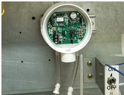
Figure 11: Duct Static Pressure (DSP) Transducer
