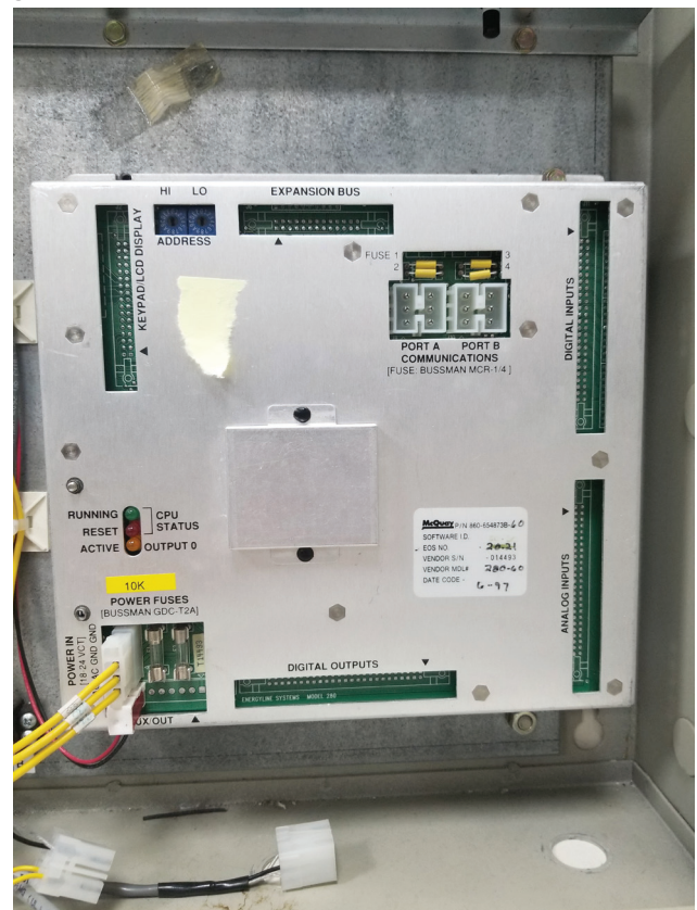
Figure 2: Main Control Board (MCB)
