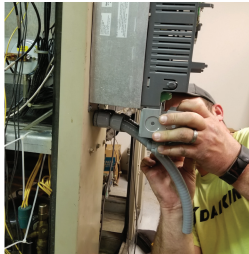
Figure 14: VFD Installed
